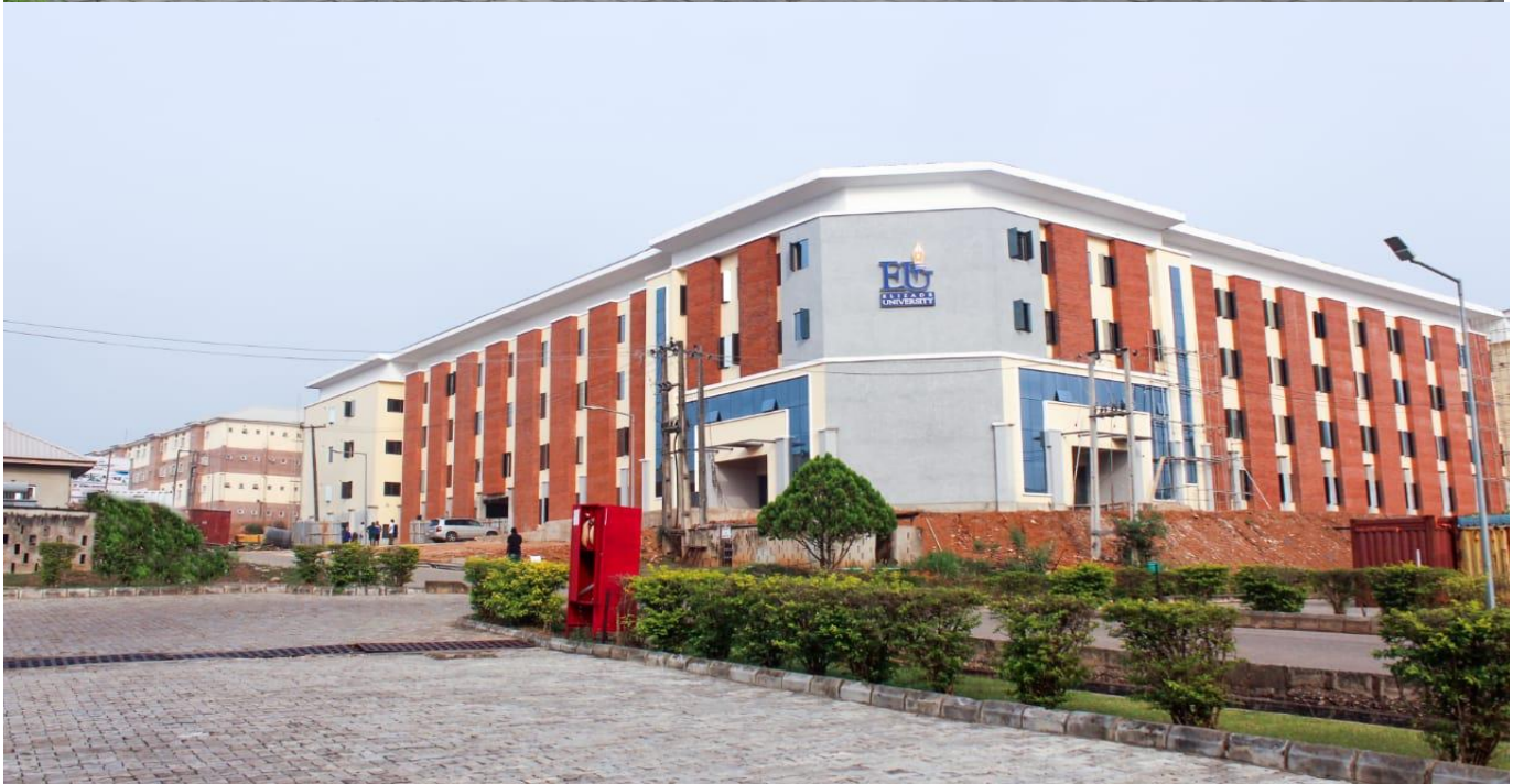
HALLS OF RESIDENCE
